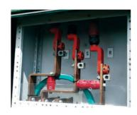
Insulated rotary clamps provide a compact connection to a slotted busbar.
